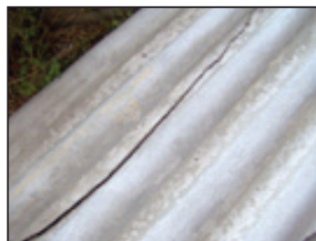
Asbestos cement roof sheets
