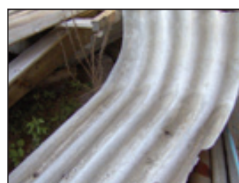
Asbestos cement roof sheets
