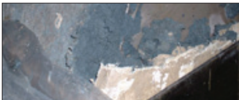
Outer cover is likely a fibreglass mixture covering the underlay of blue asbestos.
