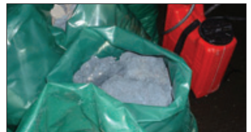
Next to the bag containing blue asbestos waste, the spray tank used to wet the asbestos lagging before stripping.
